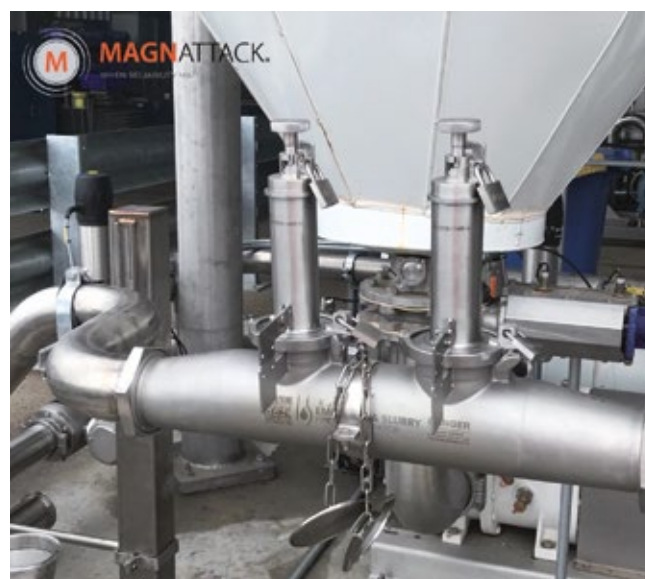
Emulsion & Slurry Pipeline Separator installed in a pet food application
