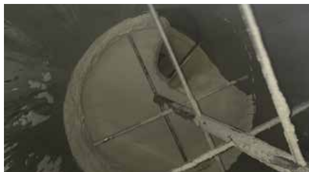
Insert Figure 1 in this section. Caption, Ratholing example
